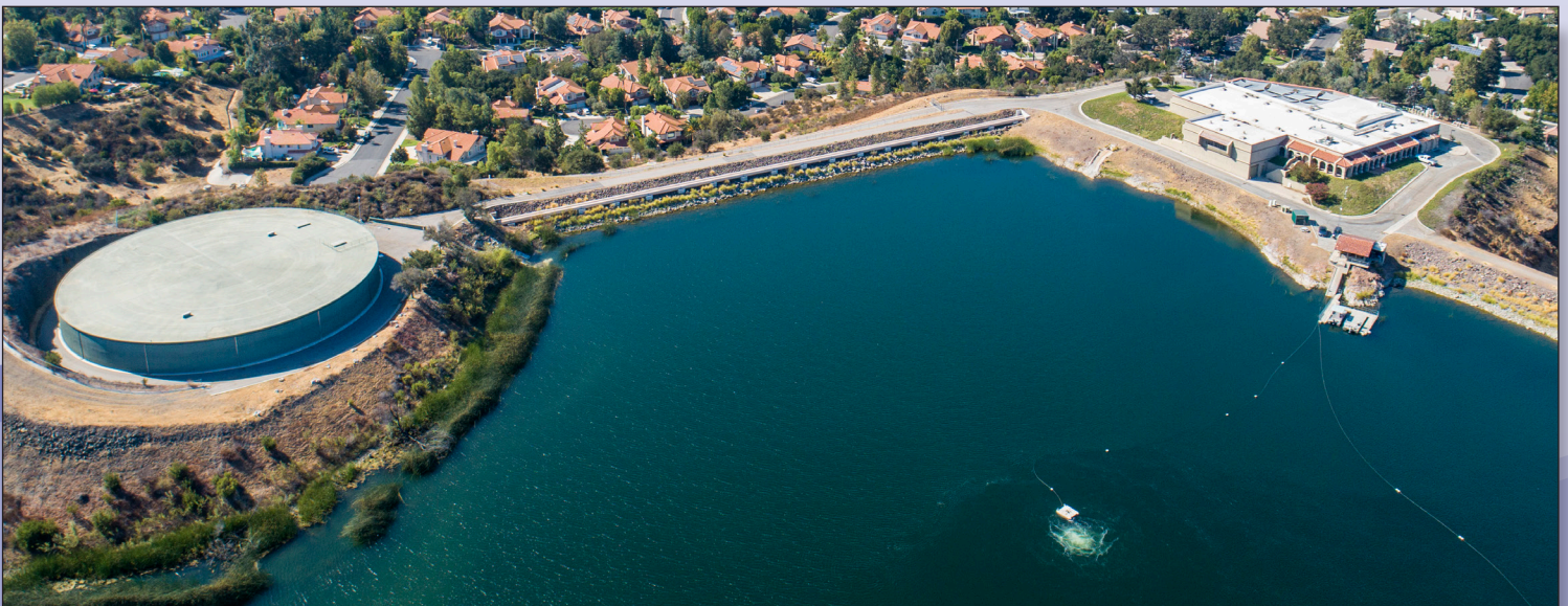
Las Virgenes Reservoir and the Westlake Filtration Plant
